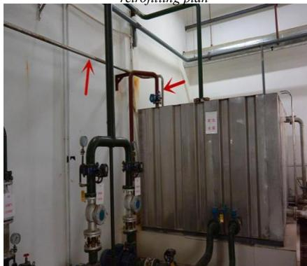
Picture 3 Soft water transfers to the water tank in boiler room
